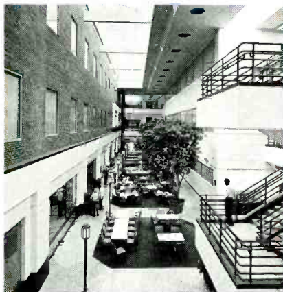
THE NEW EXPANSION OF FORD'S SCIENTIFIC RESEARCH LABORATORY was built as two building wings connected by a 40-foot, open-air atrium.
